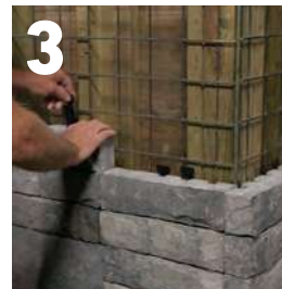
3 Attach Tandem Veneer with Connector
